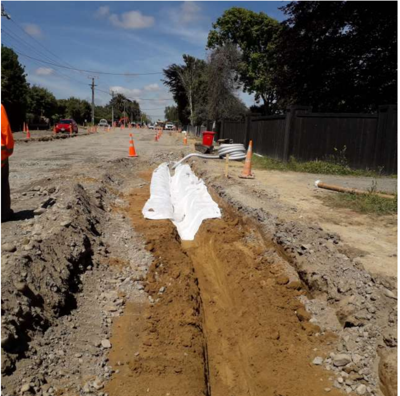
Subsoil drains being installed under kerb line (November 2017).
