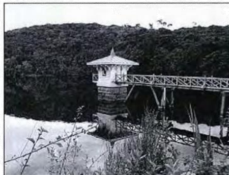
Ross Creek (No.1) Earth Dam in Dunedin (registered Category I historic place) was built in 1865 and is one of the earliest water supply dams in New Zealand.
