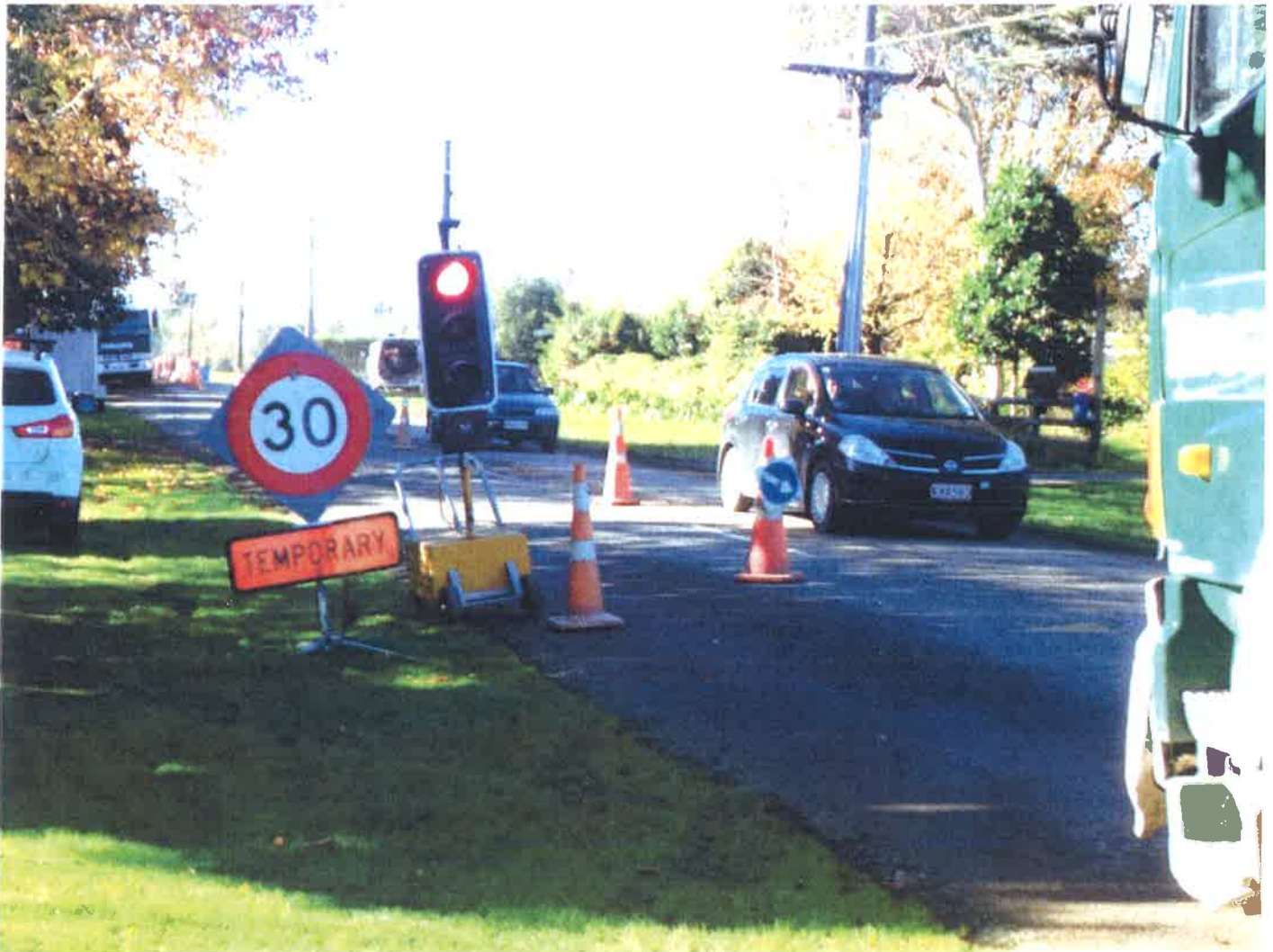
Improved Fairfield Road Traffic Management in place (May 2017).
