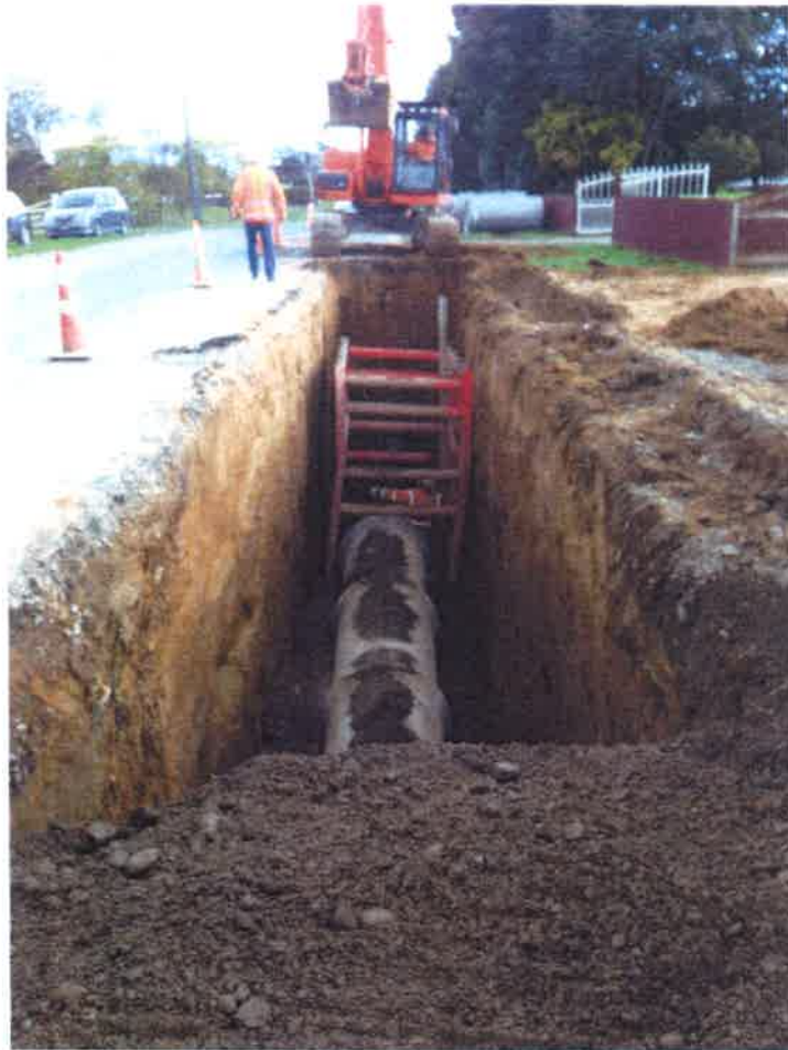
Deep trench installation (April 2017).
