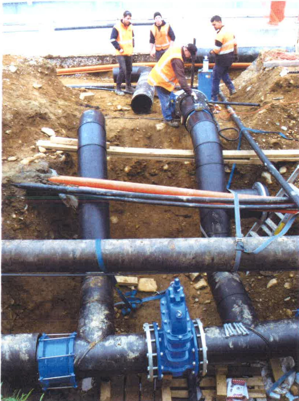
Pipe connections being completed (Apr / May 2017)
