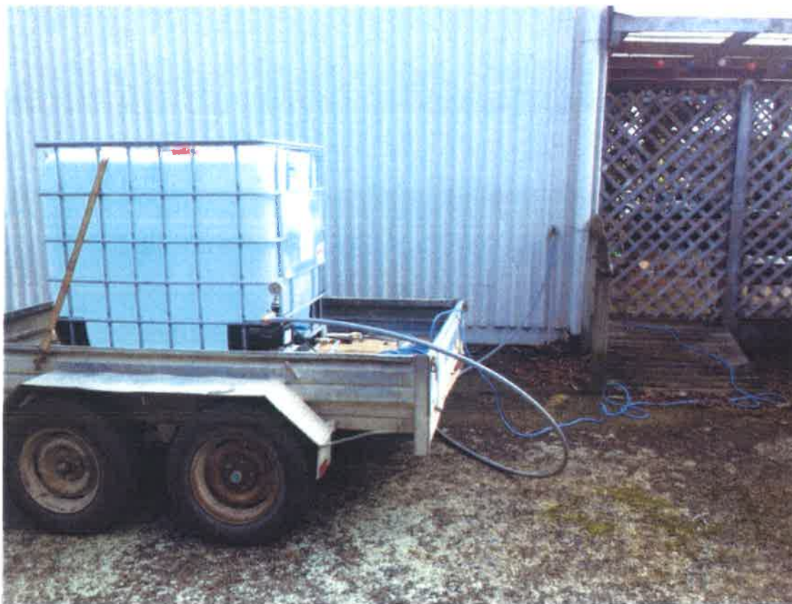
Water Tank providing temporary water supply to house with dialysis patient
