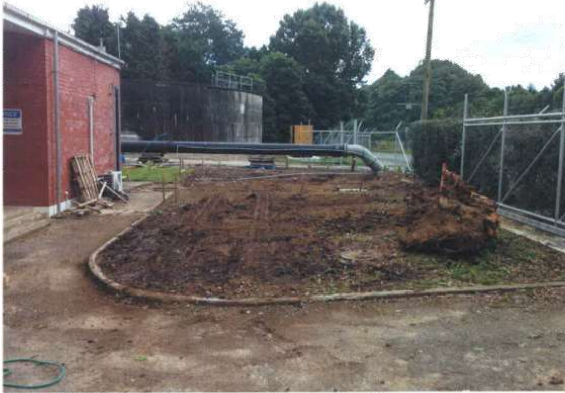
UV building earthworks (Jan 2017)
