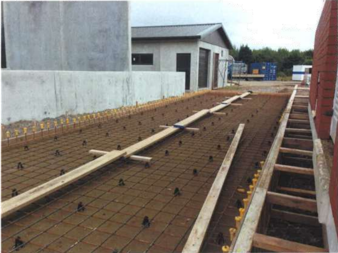
Concrete loading apron reinforcing (Jan 2017)
