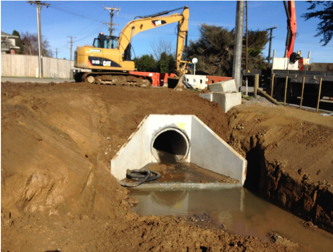
Finishing up earthworks around the relocated outlet (August 2017).
