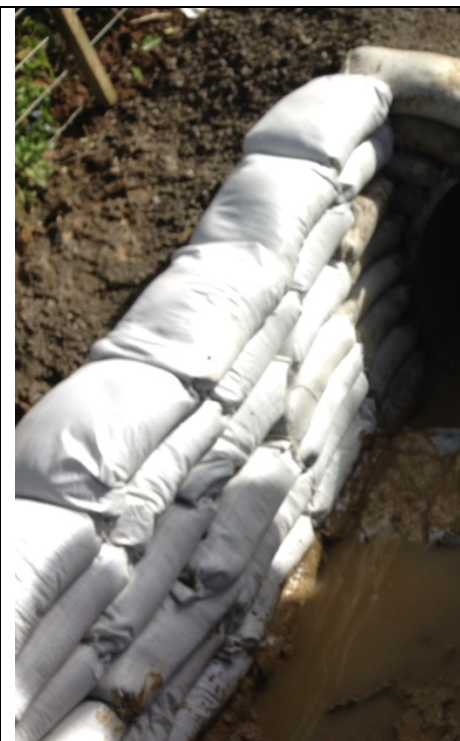
Temporary sandbags around pipe
