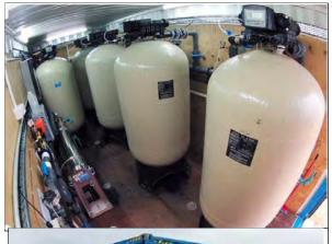
This involves the water being treated using chlorine disinfection, coarse sand filter, carbon filters, cartridge filtration and UV disinfection. The compact full-scale treatment plant was installed within a shipping container and the relatively modest project cost of just \$350,000 – less than a sixth of the original estimate – meant there was a minimal impact on rates.
