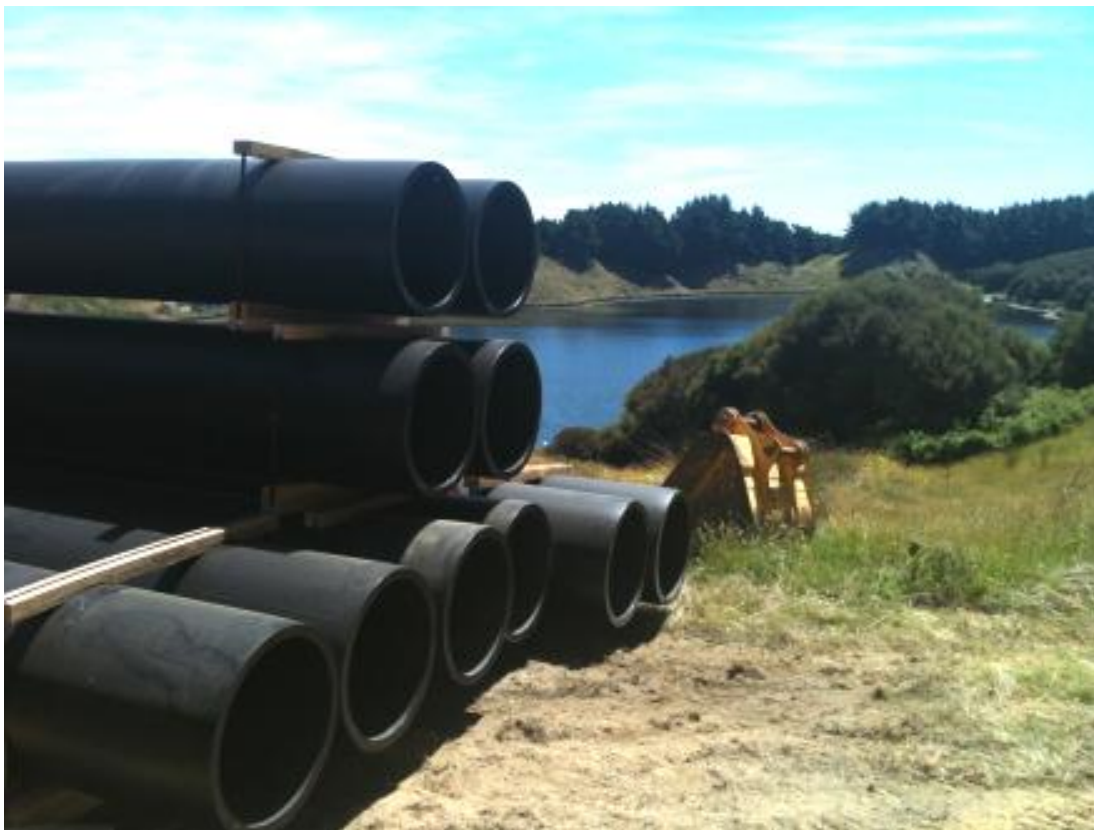
Pipes ready for installation, "Pipeline to the Pot" project, 2013
