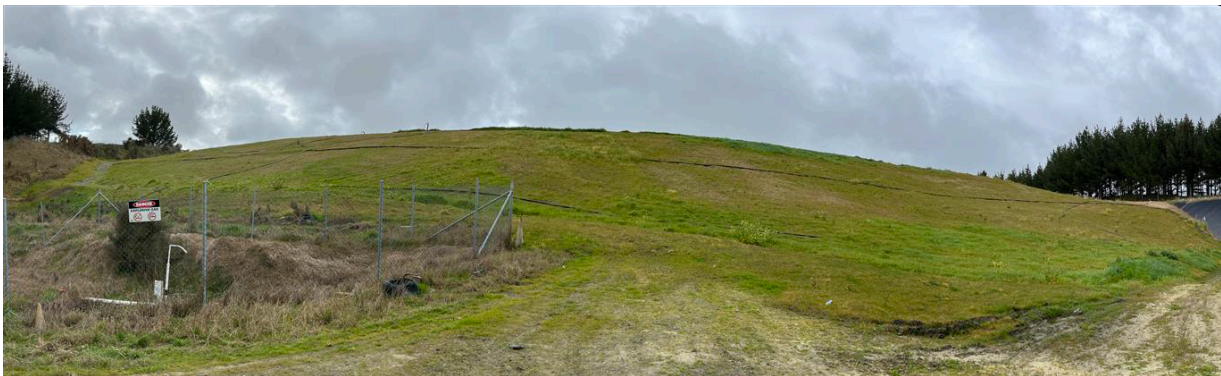
Figure 18-1: Front face of the landfill showing completed capping and vegetation.
