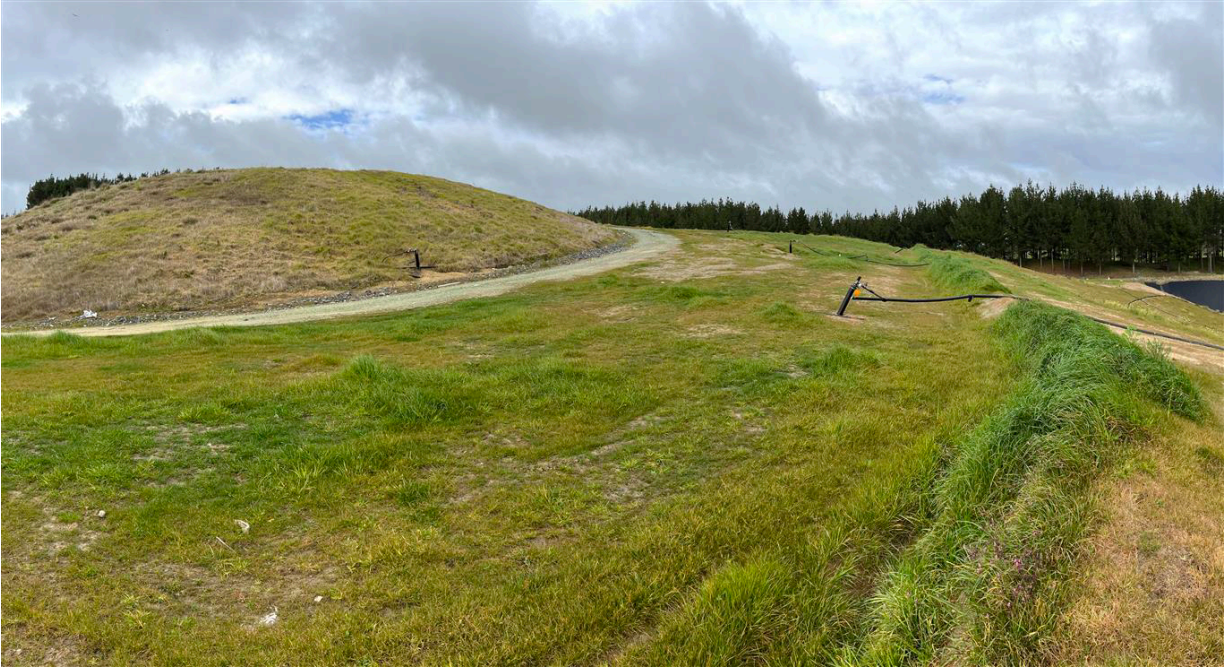
Figure 18-3: Photo showing the crest of the landfill front face slope with access road leading to the top.
