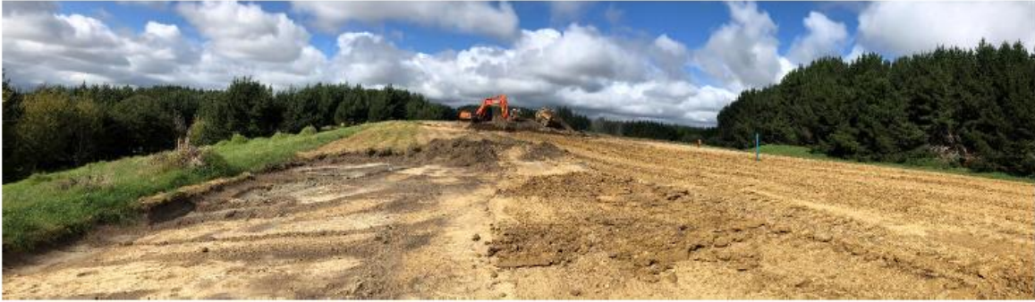
Figure 11-1 Photograph taken on 05 April 2023 showing the capping layer under construction.
