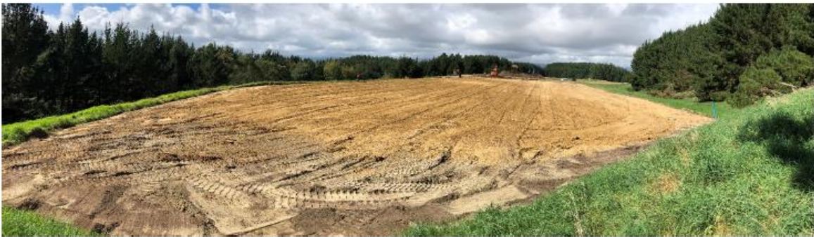
Figure 11-2 Photograph taken on 05 April 2023 showing the capping layer under construction.
