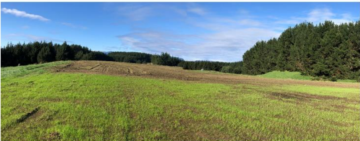
Figure 11-3 Photograph taken on 12 May 2023 showing the completed capping layer.
