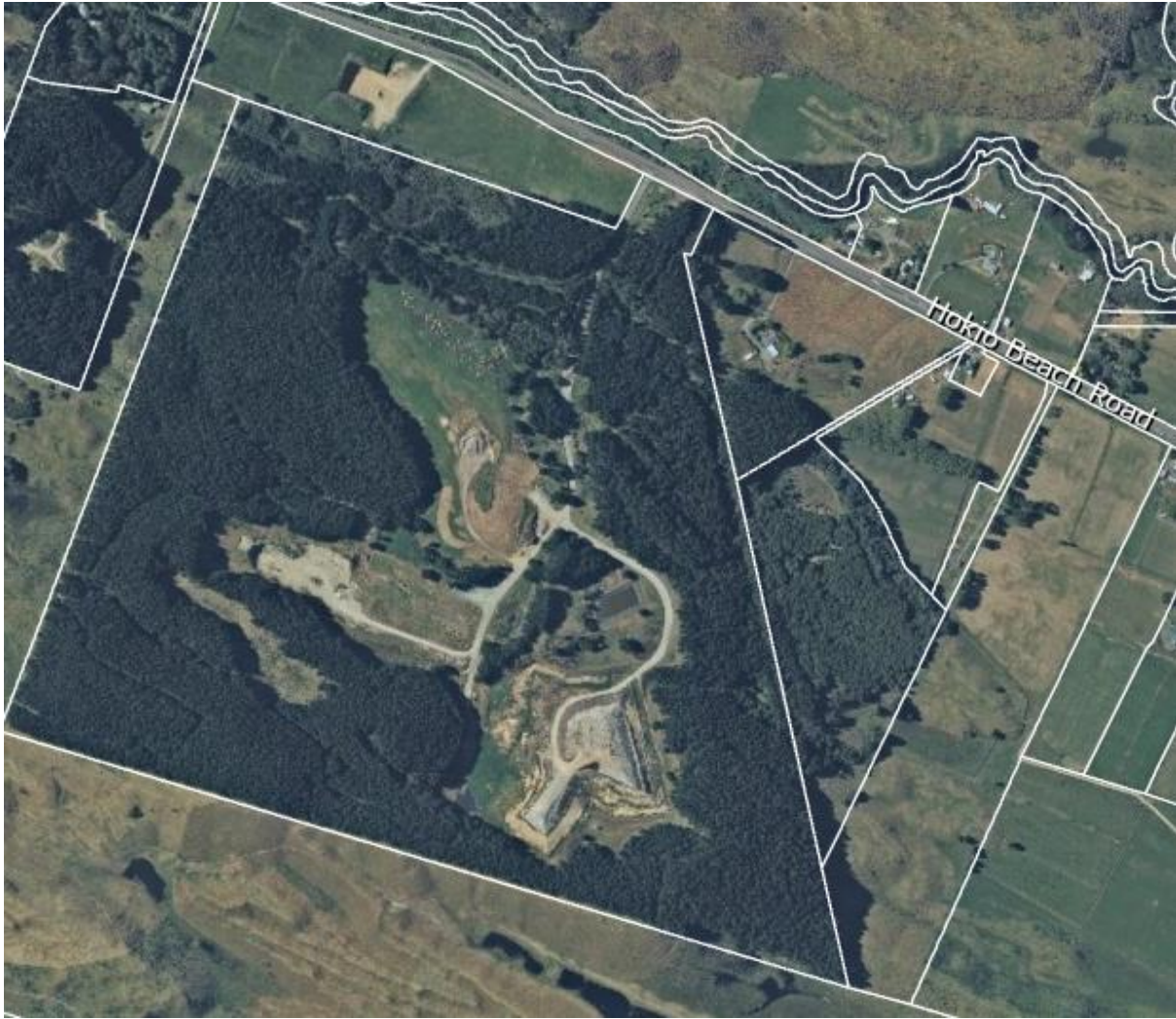
Figure 1: Aerial Photo of Levin Landfill Site
