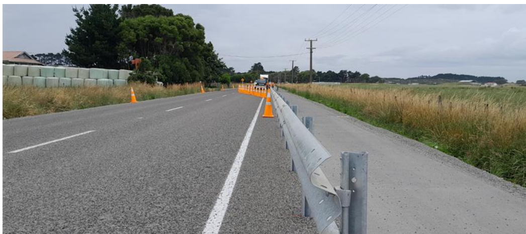
Foxton Beach Road rehabilitation works.
