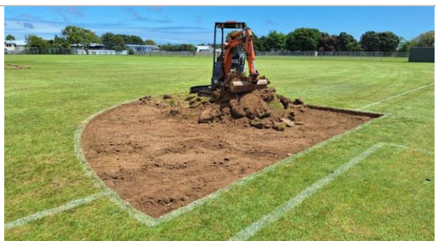
Works being done at Western Park for new clay base zones.
